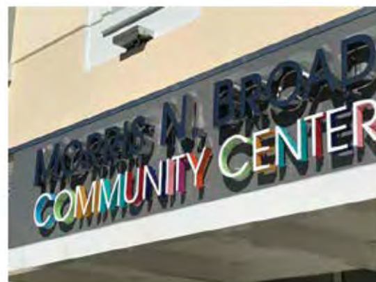
Polished stainless steel letters w/ halo illumination. Creative color used on returns of letters.
